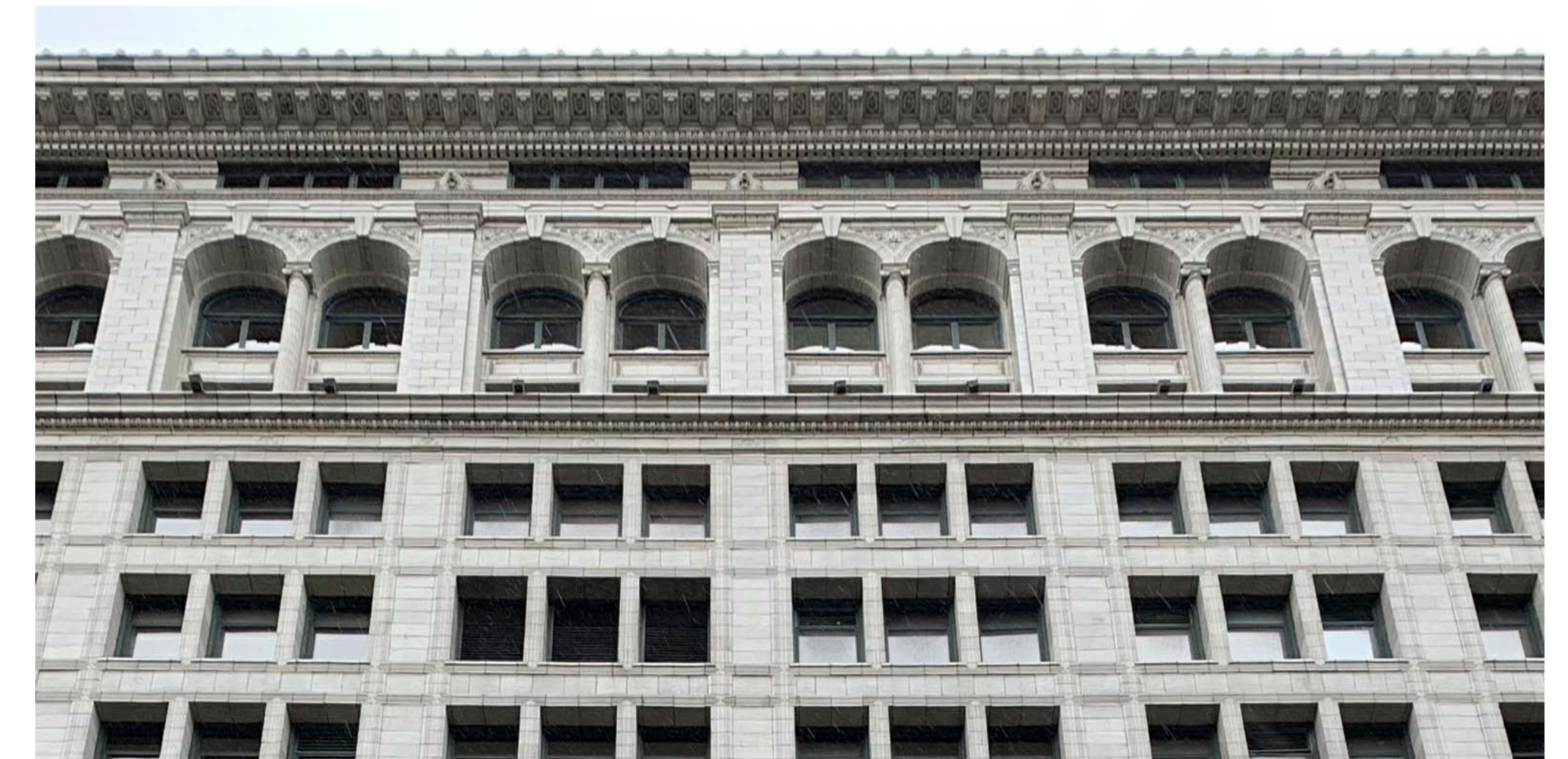
CLOSE UP - NORTH FACADE
