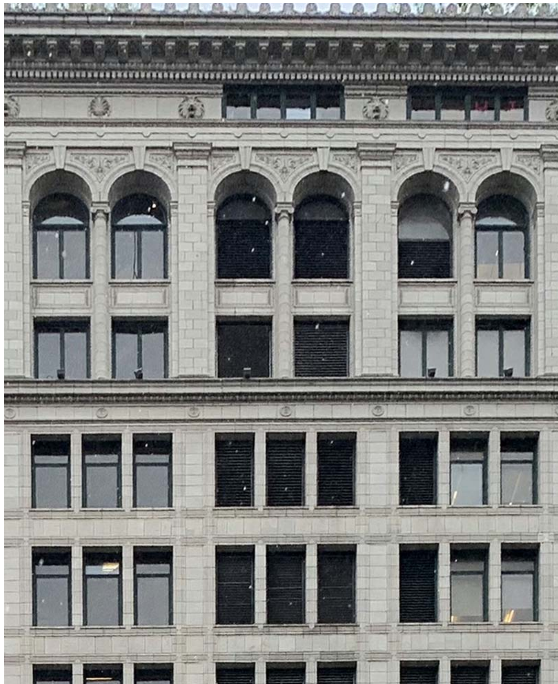
CLOSE UP - EAST FACADE
